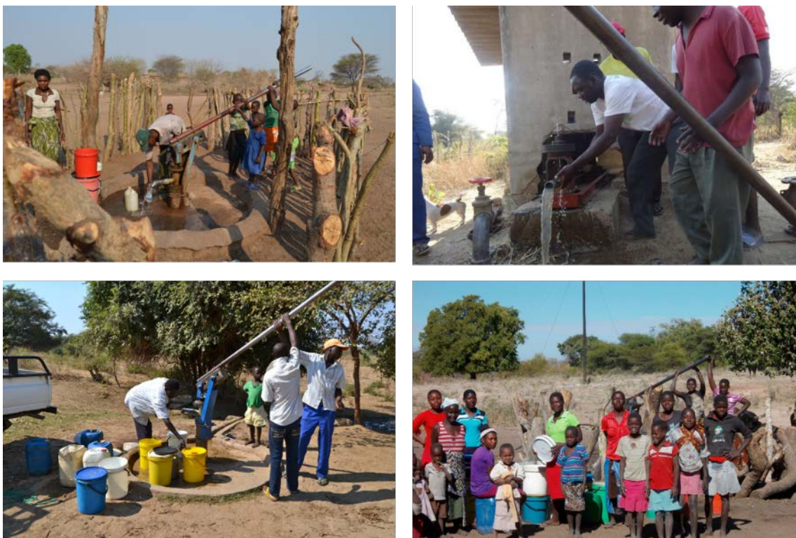
Photo 7. Borehole resuscitation and maintenance by the On the Ground Management Teams
