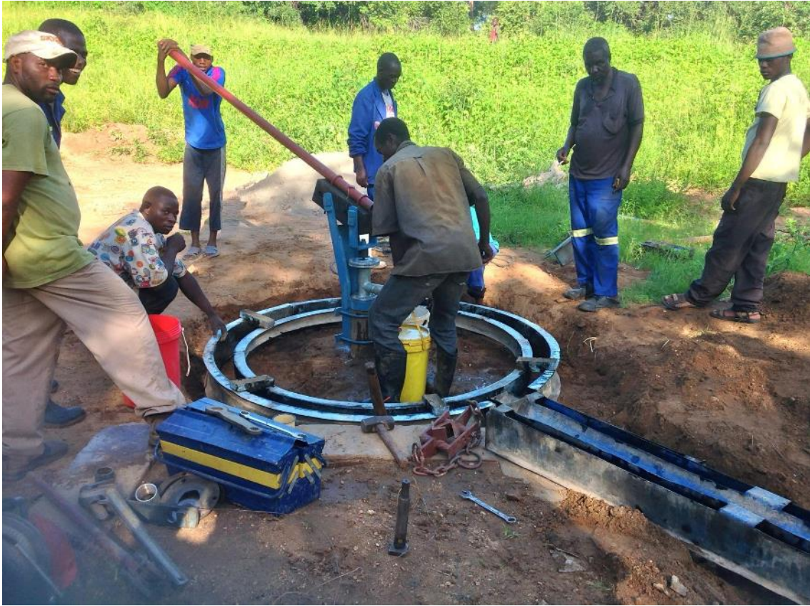
Photo 8. Borehole repair
